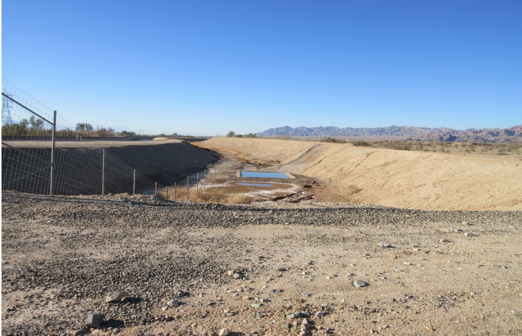
Plate 4. View of old, unlined portion of the Canal towards the north at curve in alignment south of Check 11. Note overall level of disturbance and wildlife drinker midframe. Lined canal is shown to the left.
