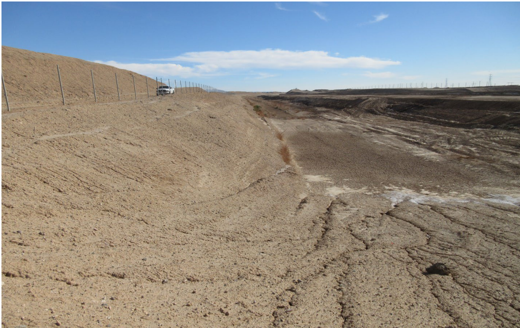
Plate 1. View along east side of original Coachella Canal towards south; embankment created from canal construction spoils shown to east.
