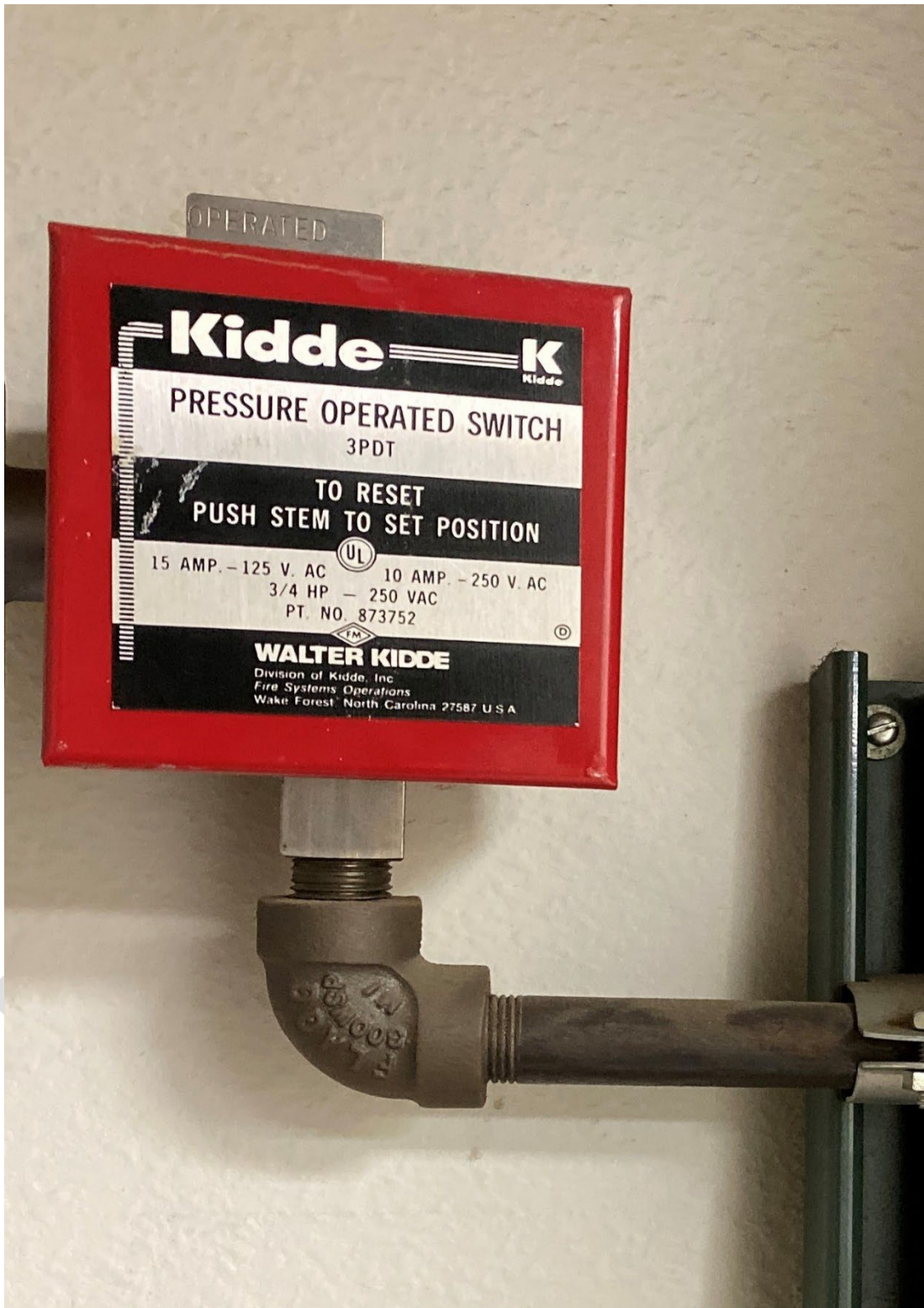
Coachella SCADA Room Halon Bottle Switch
